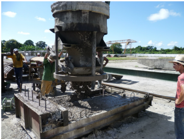
Use of LC 3 in industrial casting in Cuba
