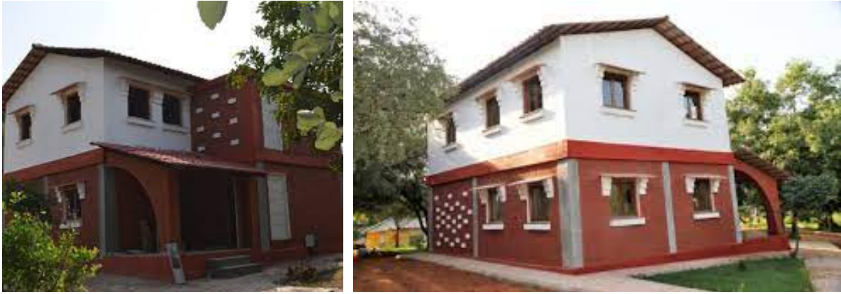
Figure: 1 a) Front view, and b) back view of LC3 building TARAgam Orchha (near Jhansi), Madhya Pradesh, India
