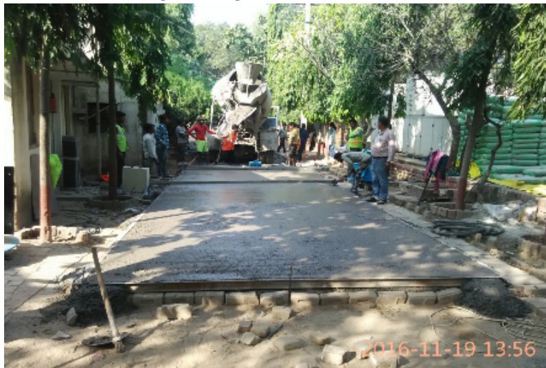
Road built at Ghitorni, New Delhi, India
