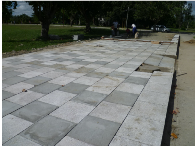
A pavement made using LC 3 in Cuba
