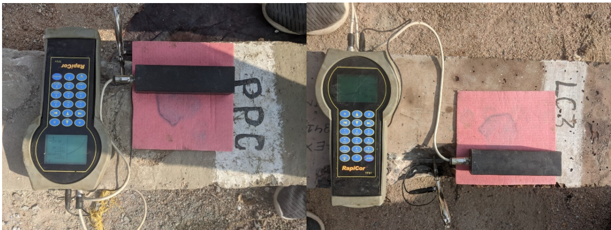
Figure: 9 Corrosion testing of PPC and LC3 columns with Rapicorr machine.
