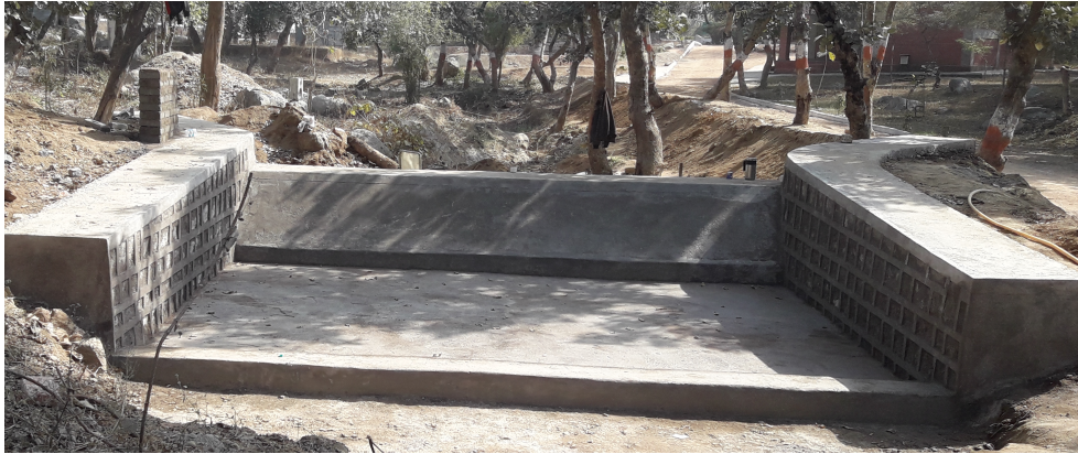
Check-dam built at Orchha by TARA
