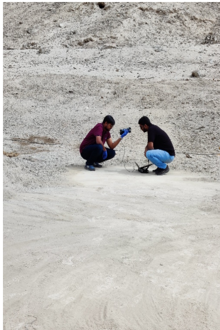
Inspection of pavement made using LC 3 in Leh, Ladakh, India
