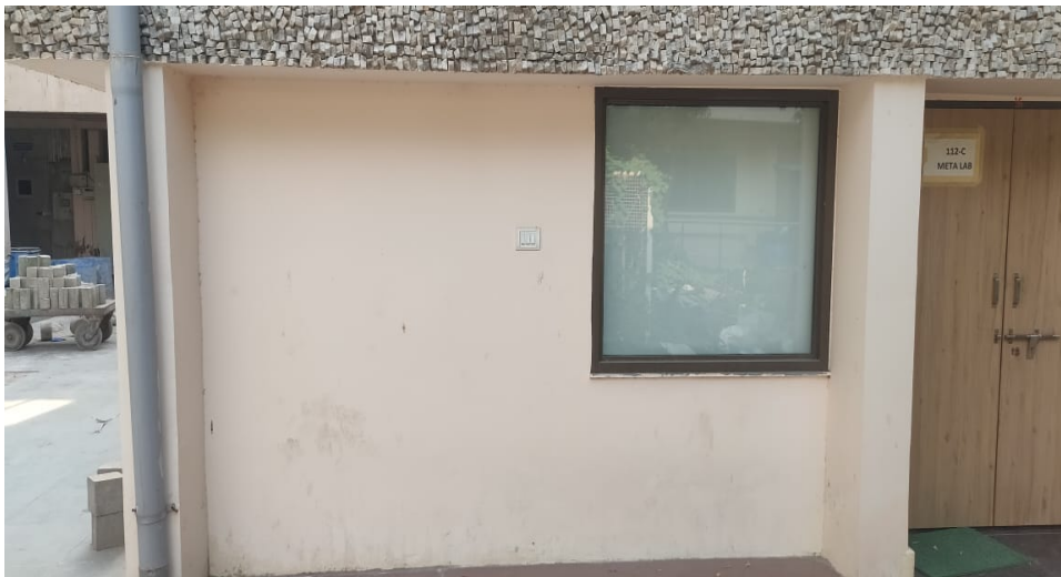
Figure 4: The current state of hardened plaster made with LC 3 cement
