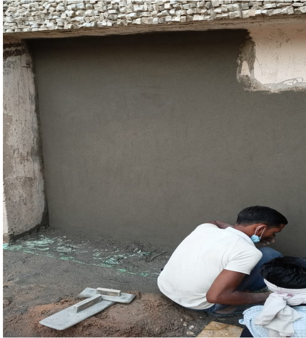
Figure 3: The finish state of the plaster on the brick wall surface.
