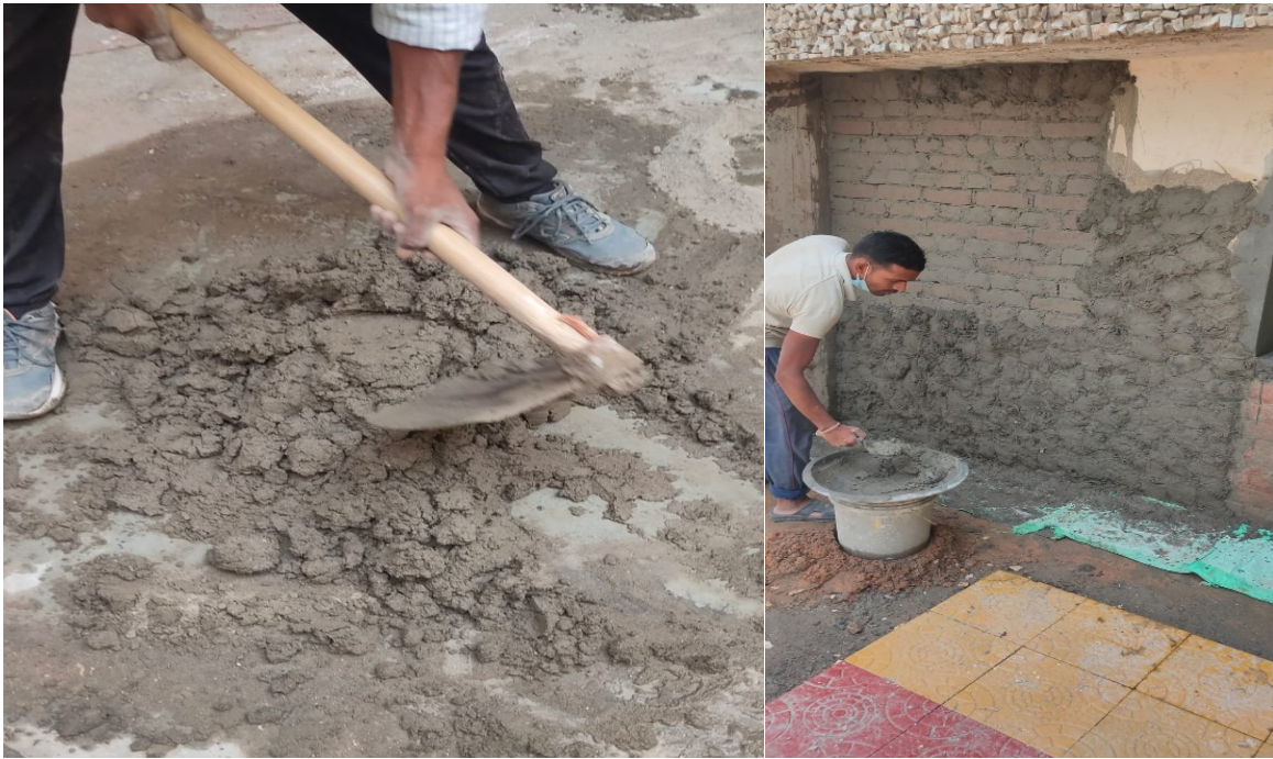
Figure 1: The picture above shows the manual mixing performed with manual labor of the plaster mix (left). The application of mortar mixes on the surface of the brick wall (right)
