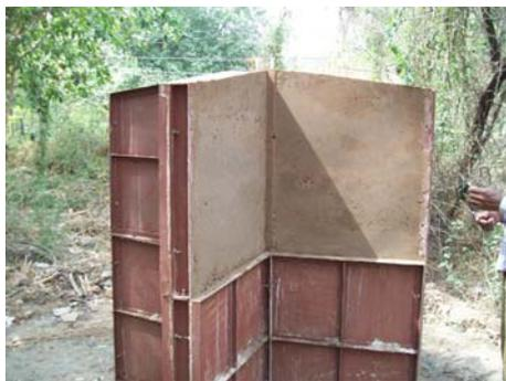
Figure8. Formwork used for fabrication of public urinal kiosk (Photo: )
