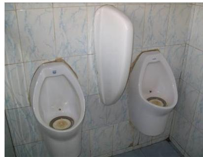
Figure 4. Urinals with sealant liquid based odour traps (Photo:R.Sakthivel)
