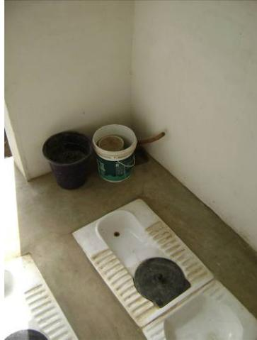
Figure15. Squatting type urine diverting dry toilet with two chambers (Photo: Dr. Lucas Dengel)
