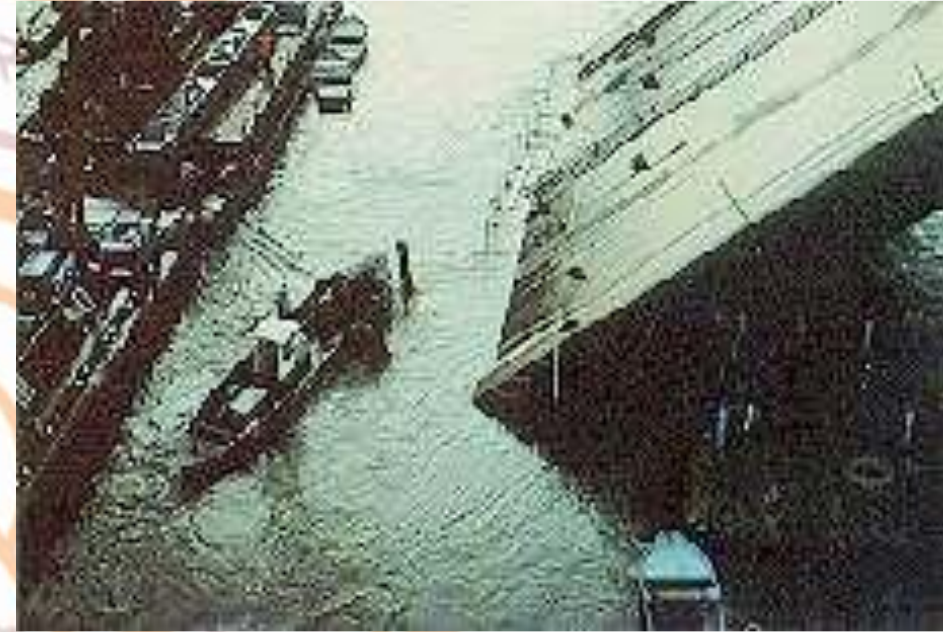
Mianus river bridge collapse in Greenwich, June 1983 (USDT, 2003)
