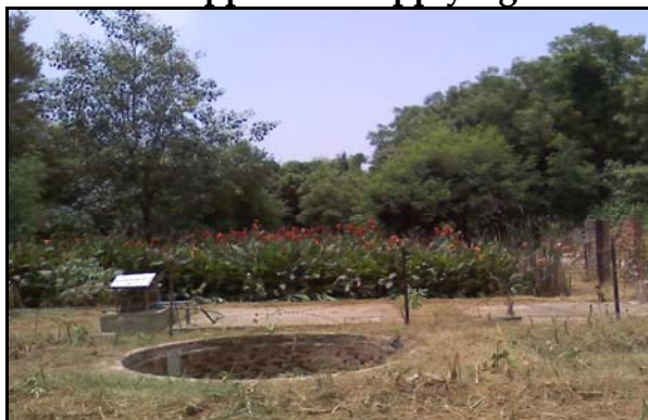
Figure 2: IIT-Delhi WWT R&D Plant
