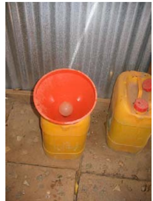
Figure14. Self constructed urinal “Eco-lily” (Source: GTZ)
