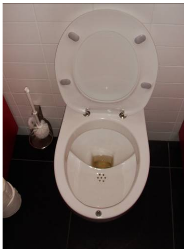
Figure16. Urine diverting no mix toilet (Source: www.washjeff.edu )
