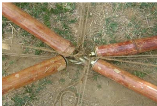
Fig 2.9. Joints used at centre of roof
