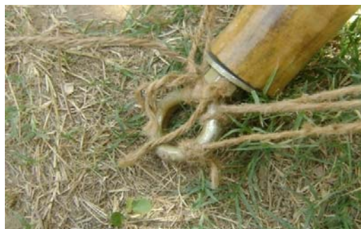
Fig 4.7 Newly Fabricated Column base joint
