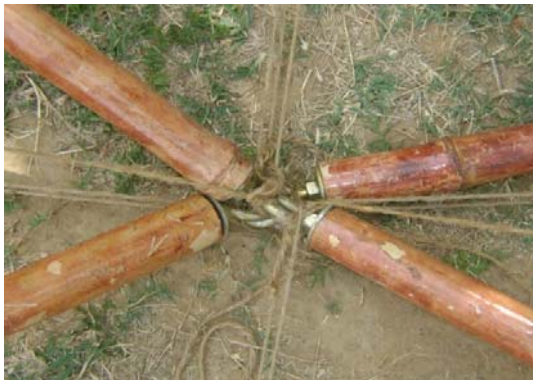
Fig 4.5. Newly Fabricated Central Roof Joint
