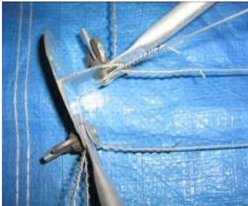
Fig 4.3: Previously used joint in the middle of Roof base Source: Goyal A (2008)
