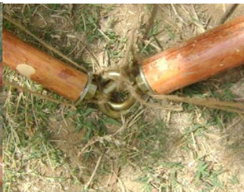
Fig 4.6. Newly Fabricated joint used in the middle of the roof base
