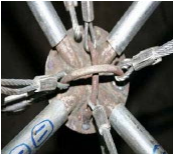
Fig 4.1: Previously used Circular-plate joint Source: K. Vijay Kumar(2007)
