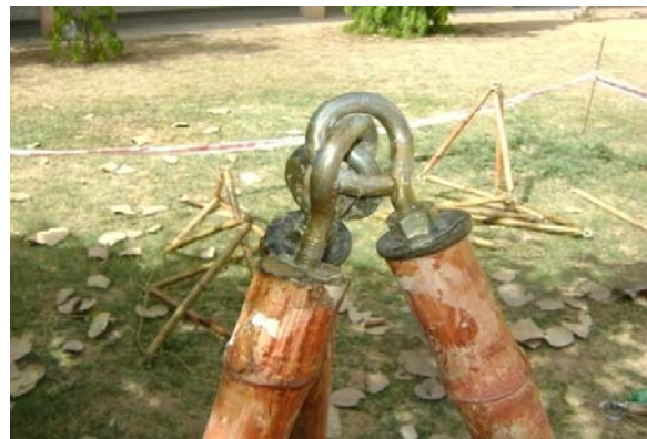
Fig 2.4 Joint used for connecting column to roof
