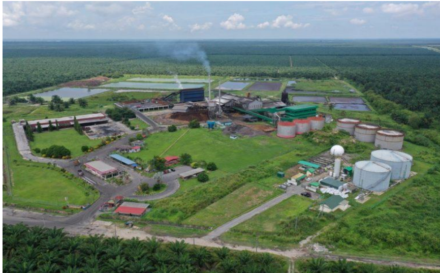
Fig. Seberang Perak biogas plant. The plant sits on the site of the palm oil mill from which BiON will take the palm oil mill effluent (POME) to generate electricity to be fed into the national grid. (Source: Bioenergy Insight)
