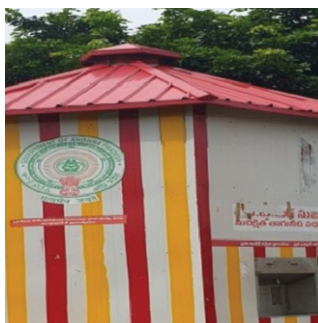
CONSTRUCTION OF R.O. PLANT IN PATHAVARAKA VILLAGE
