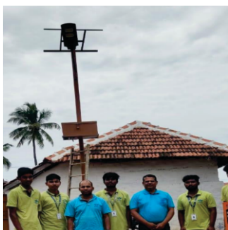
INSTALLATION OF INTEGRATED SOLAR LIGHTS
