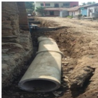
DEVELOPMENT OF UNDERGROUND DRAINAGE SYSTEM
