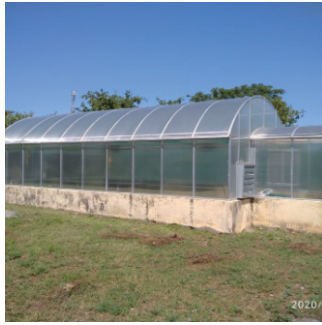
MODEL NURSERY CONSTRUCTION
