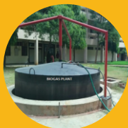
Rural Energy Systems
