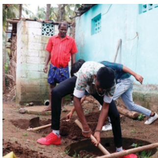
RENOVATION OF TOILETS IN PUTHUPATHI TRIBAL VILLAGE
