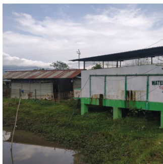
9000 L WATER TREATMENT PLANT BASED ON ROUGHING AND BIOSAND FILTERS
