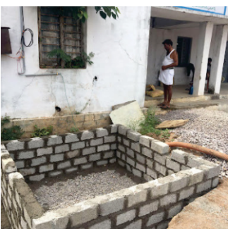
RAIN WATER HARVESTING PITS
