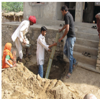
SOAK PIT CONSTRUCTION
