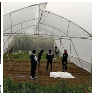
CONSTRUCTION OF POLYHOUSES
